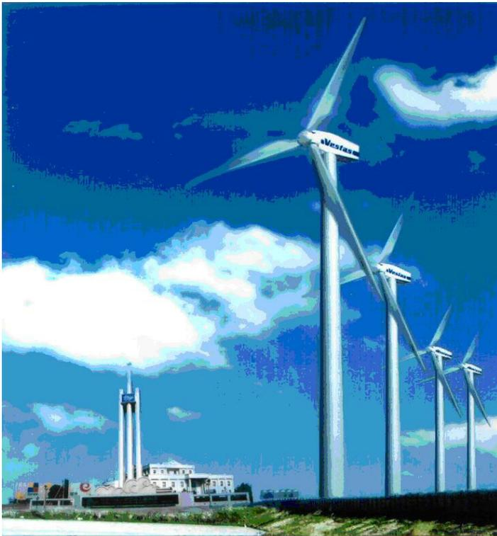
Wind turbines feature a number of components, including blades, a shaft, a generator and a tower. The blades look like propellers, except that instead of creating wind, they catch the wind. The shaft is connected to the blades, and it rotates as the blades turn with the wind. The generator transforms the rotations of the shaft mechanical energy into electrical energy.
